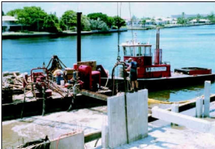
Construction on the the nine-slip marina, 23' to 46', is now complete.
