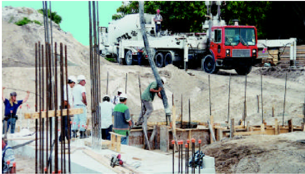
Construction workers completing installation of Mediterranea's intracoastal building foundation.
